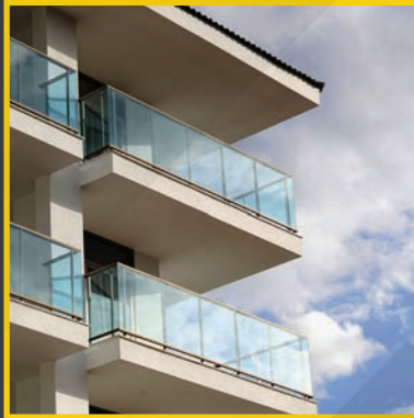
Building Construction Bauindustrie
