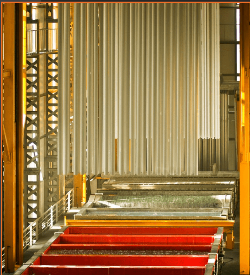
Surface Treatment Unit
