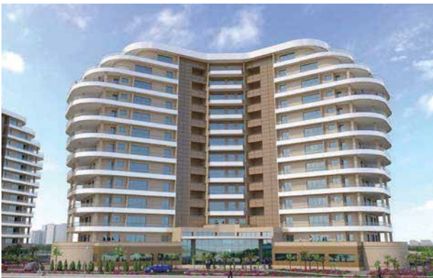
● PARSIS APARTMENT BUILDING PROJECT / IRAN
