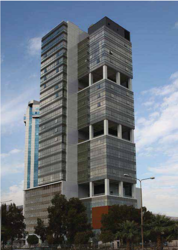
● MEGAPOL TOWER / IZMIR, TURKEY
