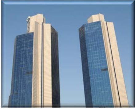
Sabancı Center – İstanbul, 1991
