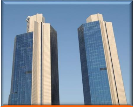
Sabancı Center – İstanbul, 1991
