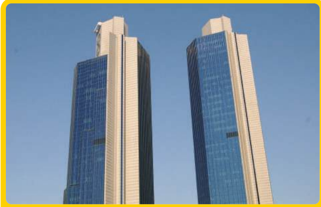
Sabancı Center – İstanbul, 1991
